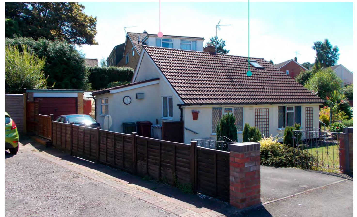
③ North West view of existing
