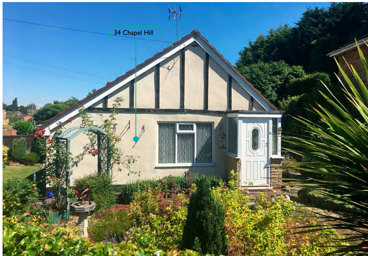
① South view of existing property
