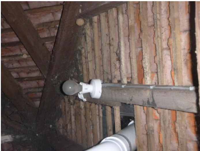
Plate 11. General view of the internal void space.
