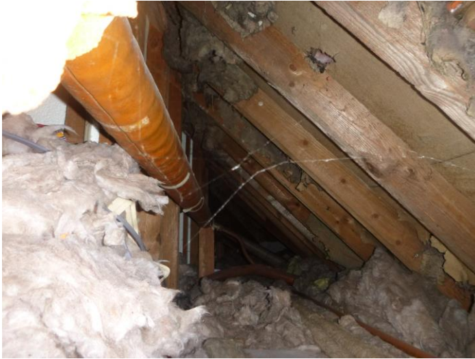
Plate 10. General view of the internal void.
