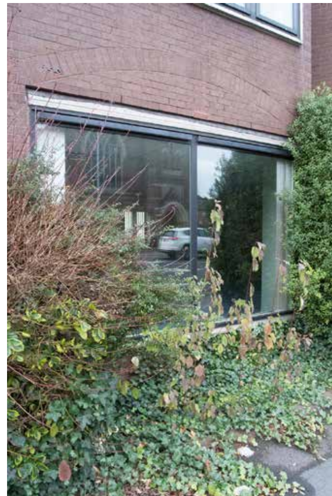
2. Ground floor south facing window
