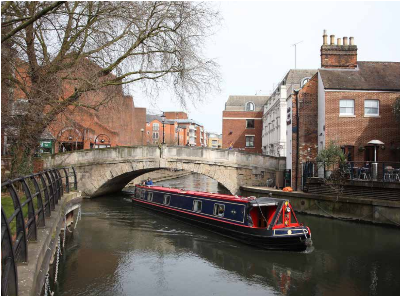
View of Duke Street Bridge along the River Kennet
