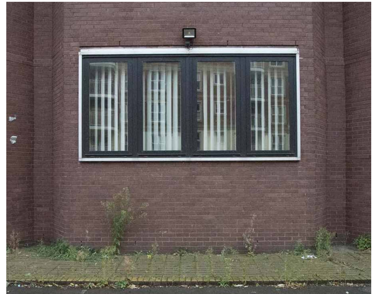
3. Typical window image shows north facing raised ground floor
