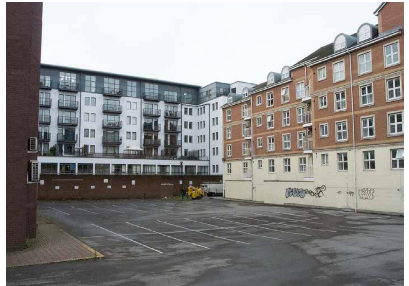
View north-west across the car park to the north of Clarendon House
