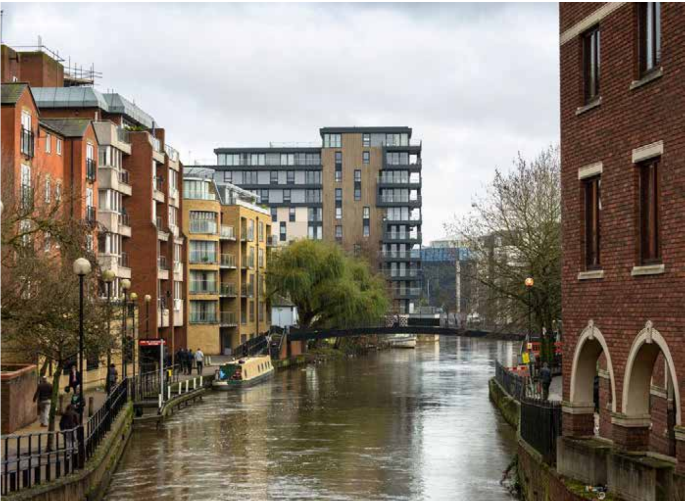
View East along the Kennet with Kennet House in the background
