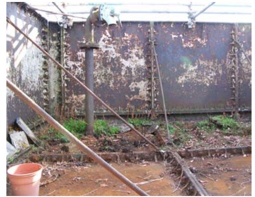
Figure 14: Interior of the cast iron tank
