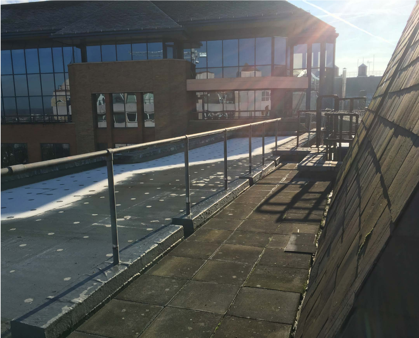
Forbury Court Roof
