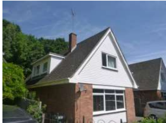
4. Roof tiles tightly fitted; second elevation clad with UPVC.
