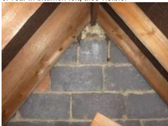
10. Fibreglass filling gaps between blockwork at gable ends.
