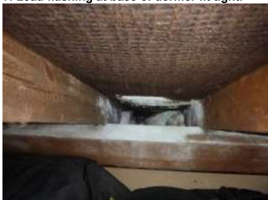
9. Styrofoam and fibreglass lining eaves
