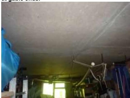
11. Roof space of garage partly-boarded centrally.
