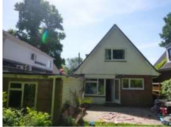
2. Rear elevation viewed from the north.
