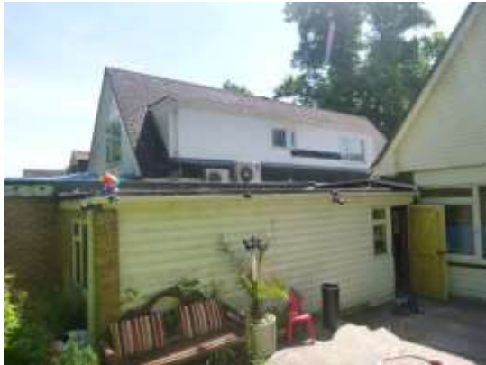
3. Rear garage extension.
