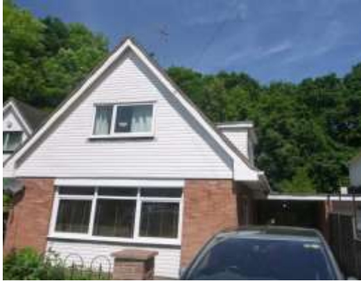
1. Front elevation viewed from south.
