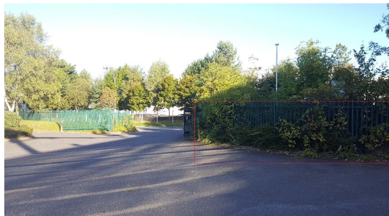
Photo 6 – Area for additional hard standing in rear service yard
