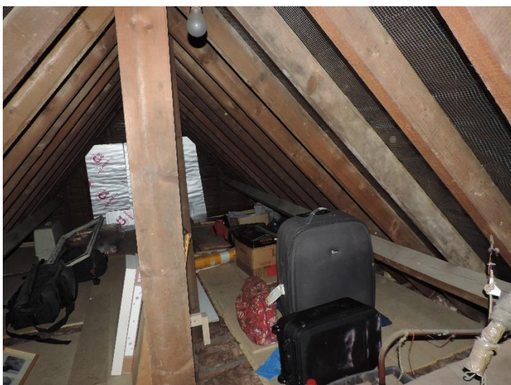
Plate 9. General view of the internal void space.
