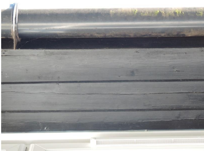
Plate 6. General view of the soffit and fascia.
