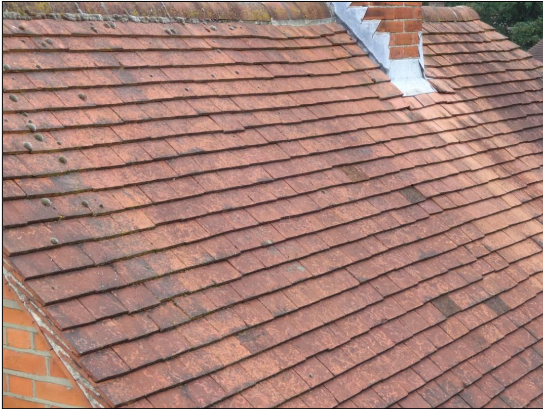
Figure 7. Example of the lead flashing, 6 Maple Gardens, Reading. 29.05.18
