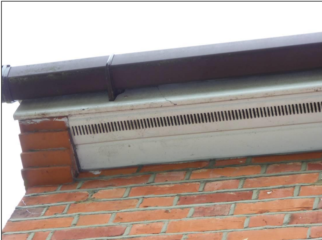
Figure 8. Fascia's and soffits, 6 Maple Gardens, Reading. 29.05.18
