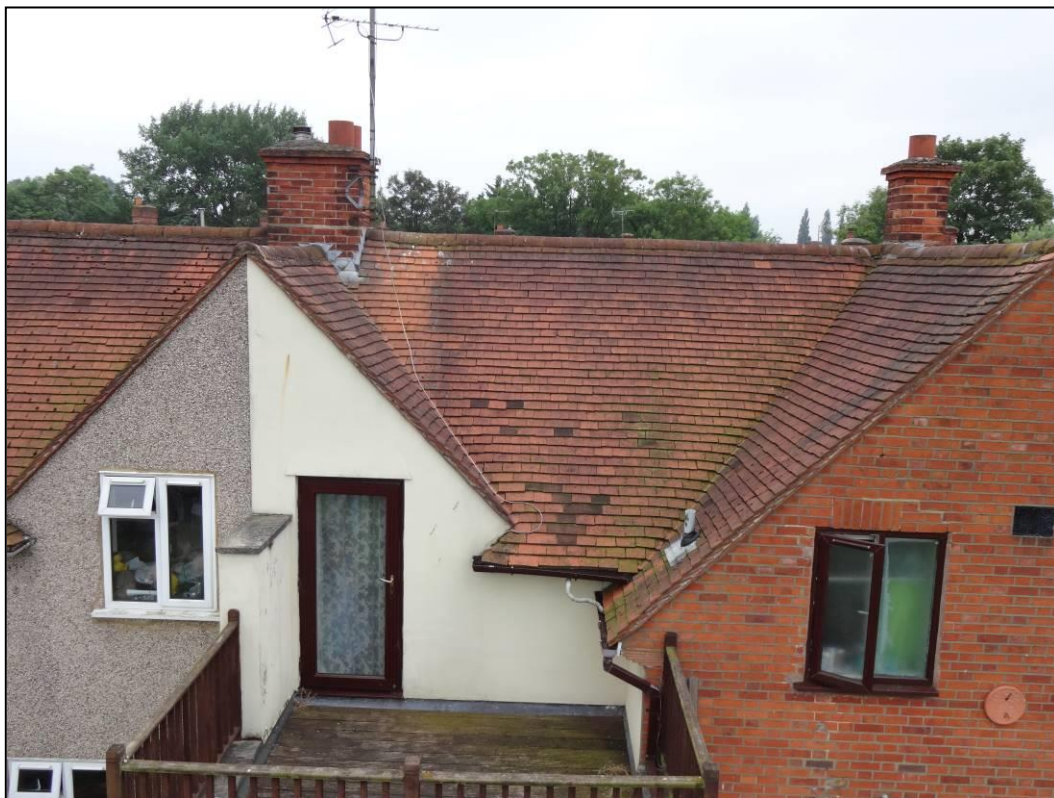
Figure 4. Example of roof structure, 6 Maple Gardens, Reading. 29.05.18
