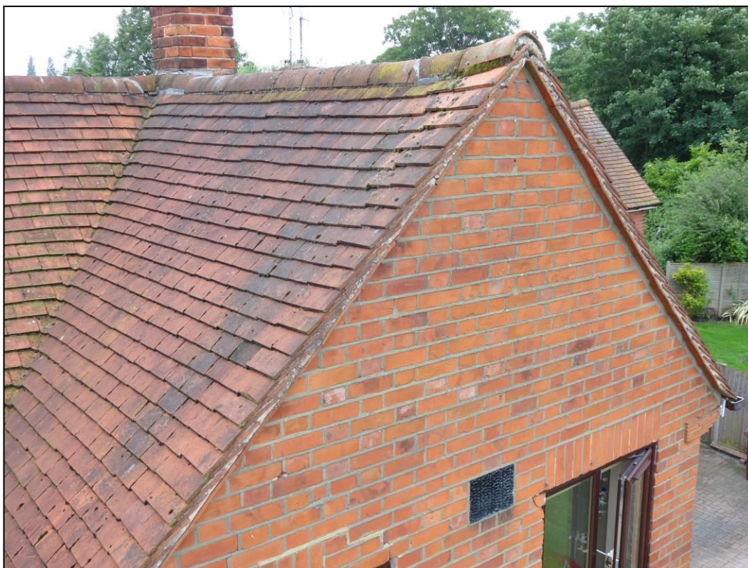
Figure 6. Verges and ridge tiles, 6 Maple Gardens, Reading. 29.05.18
