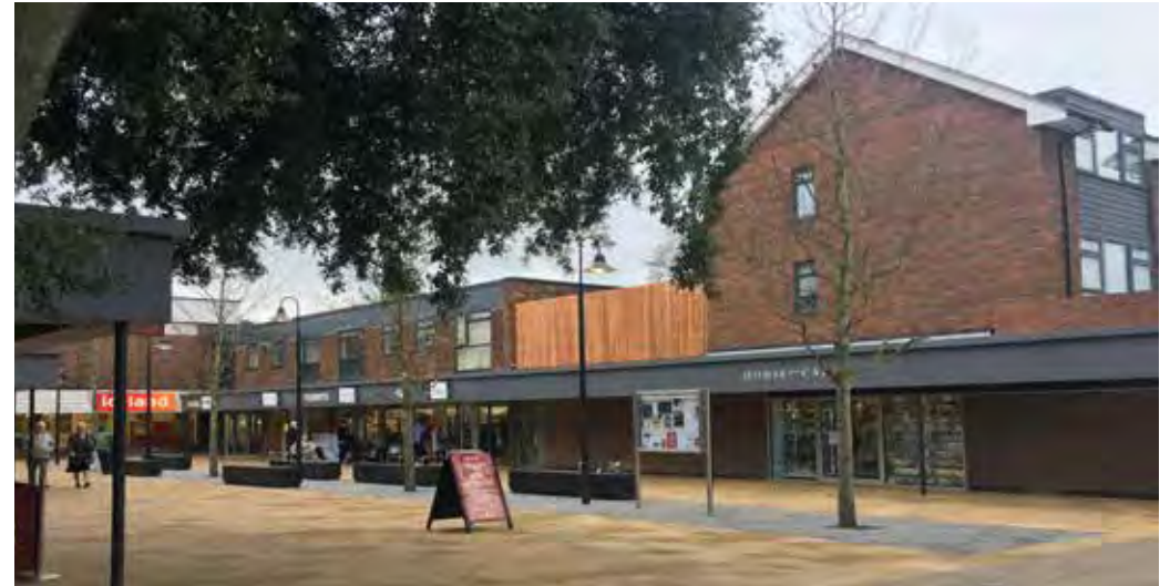
fig. 10 Recently Refurbished St Martin's Square Precinct Phase 1b
