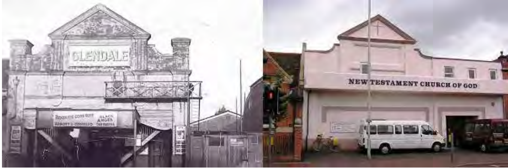
fig. 4 Site of former Glendale Cinema on Church Street
