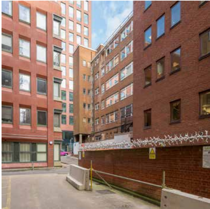
Access Road from Icon House
