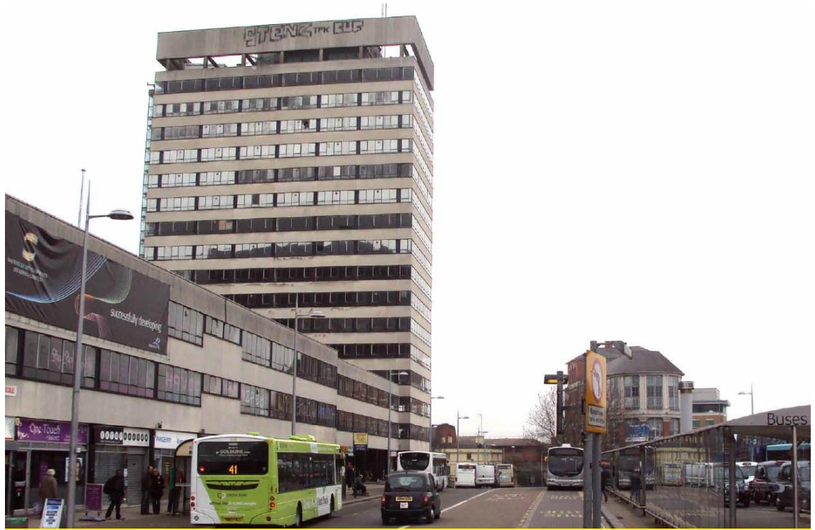
Figure 13: Photo of former western tower (17 storeys)
