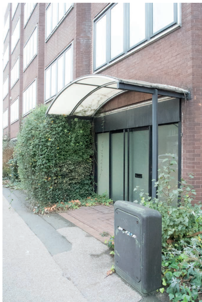
1. Entrance doors and canopy
