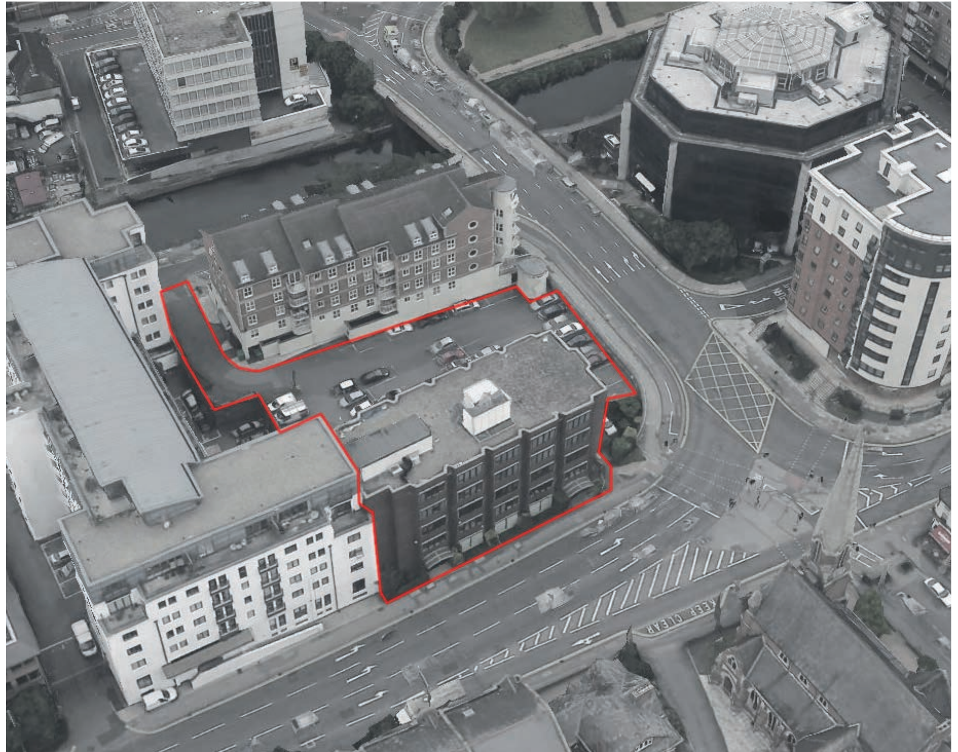
Aerial View of the Site Looking North
