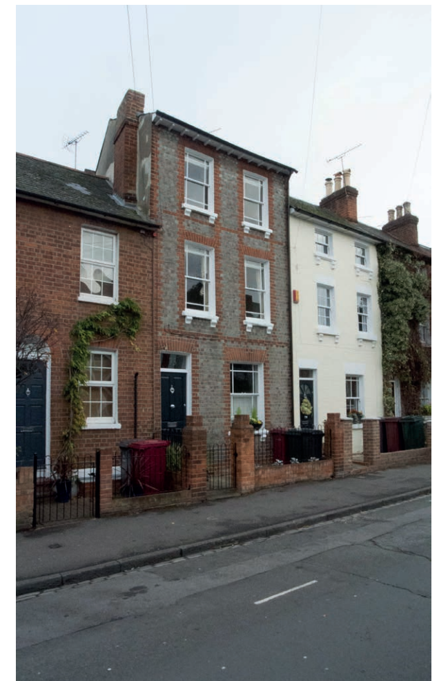
Terraced Housing Watlington Street
