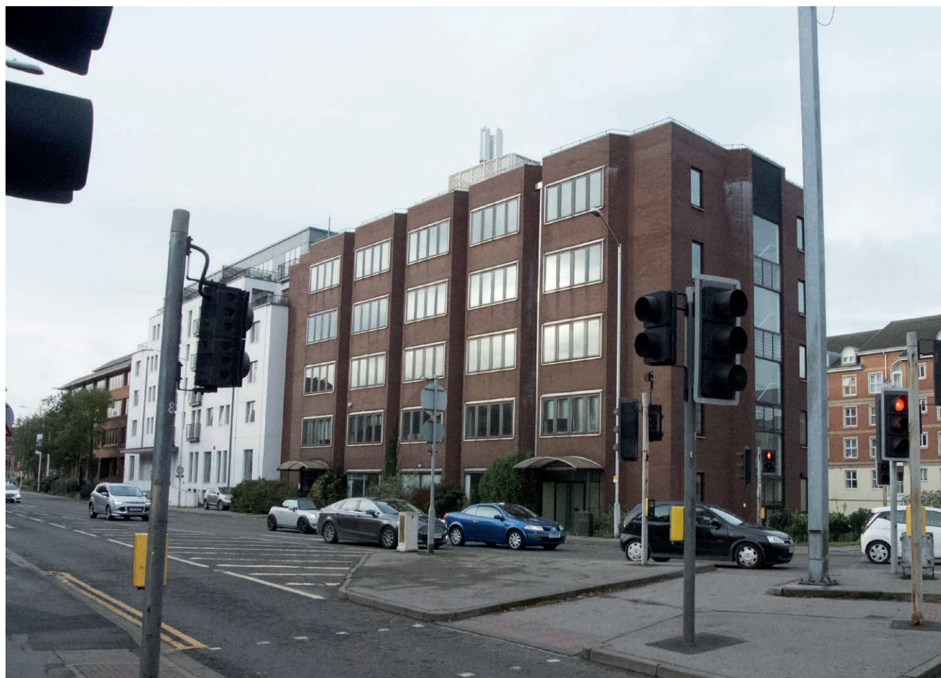
Clarendon House view towards the north-west
