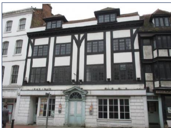
Figure 7 – 29 – 31 Market Place (Former Cooper's Arms)
