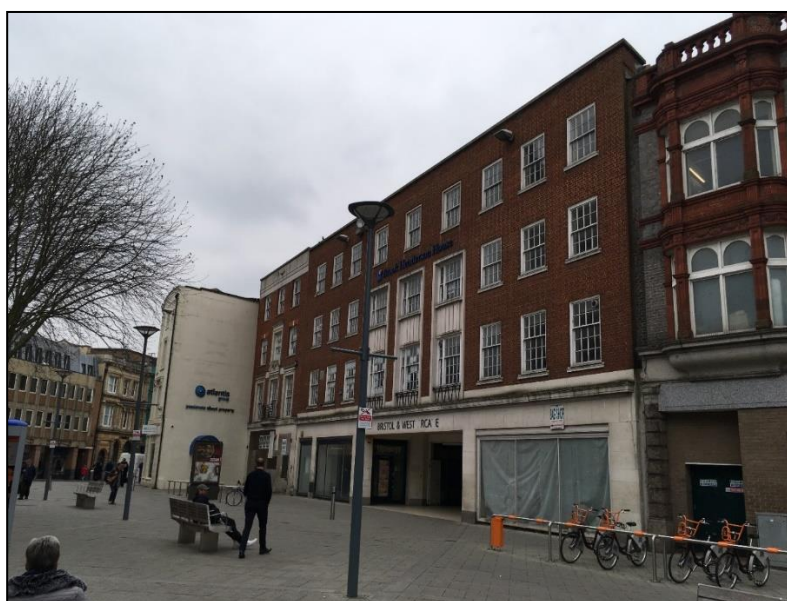
Figure 36 – Existing Friar Street elevation in March 2016
