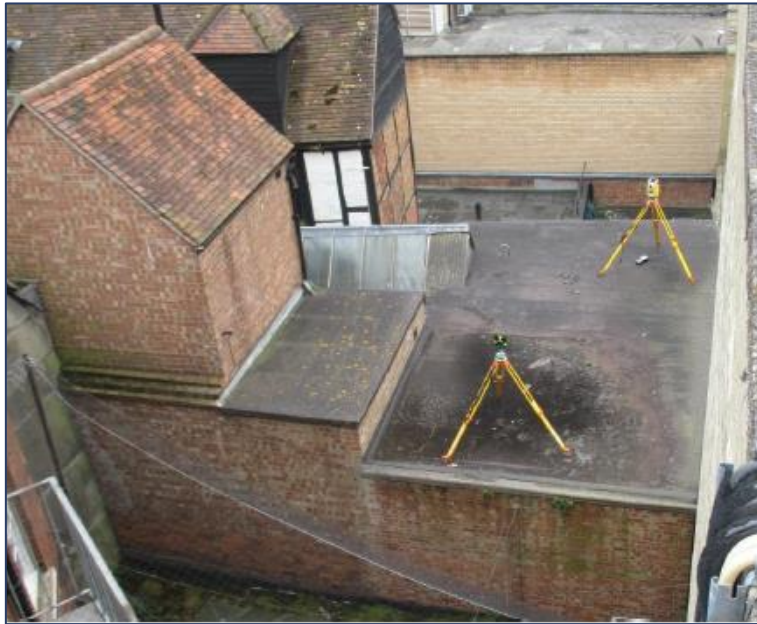
Figure 35 – Modern rear extensions to 29 – 31 Market Place
