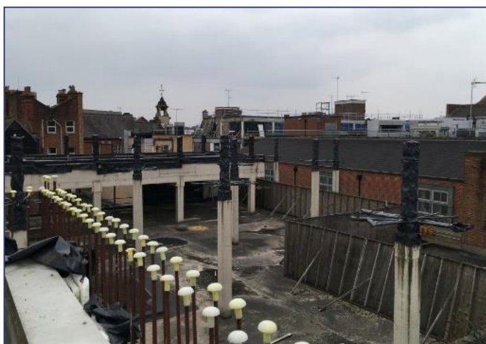
Figure 15 – Construction works to the rear of the arcade
