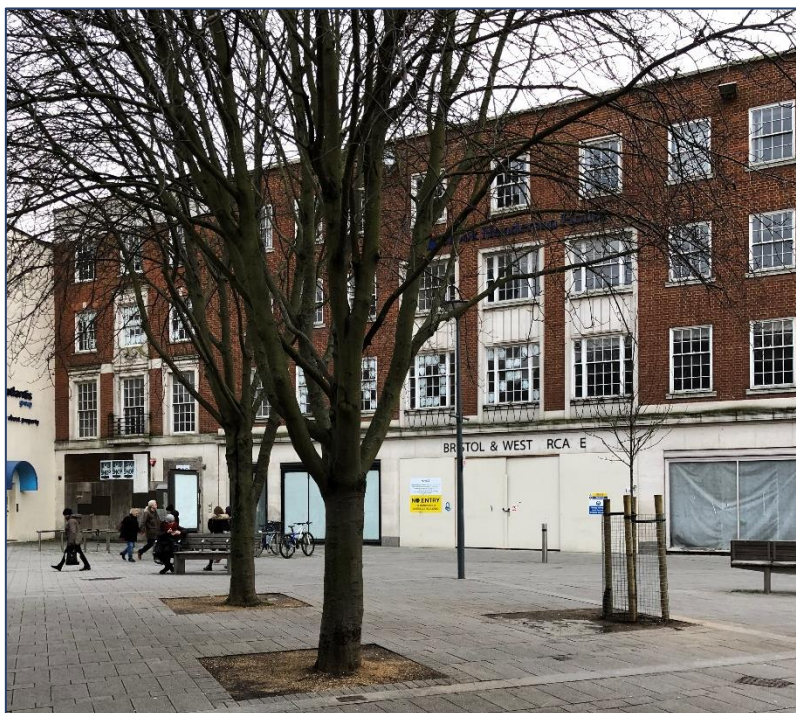
Figure 4 – Existing Friar Street building
