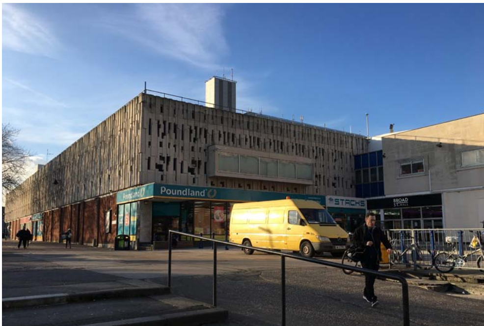
VIEW OF ADJACENT RETAIL UNIT WITH CAR PARK ABOVE
