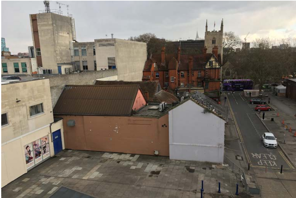
VIEW OF SOUTH COURT LOOKING EAST WITH HOSIER STREET AND ST MARYS MINSTER
