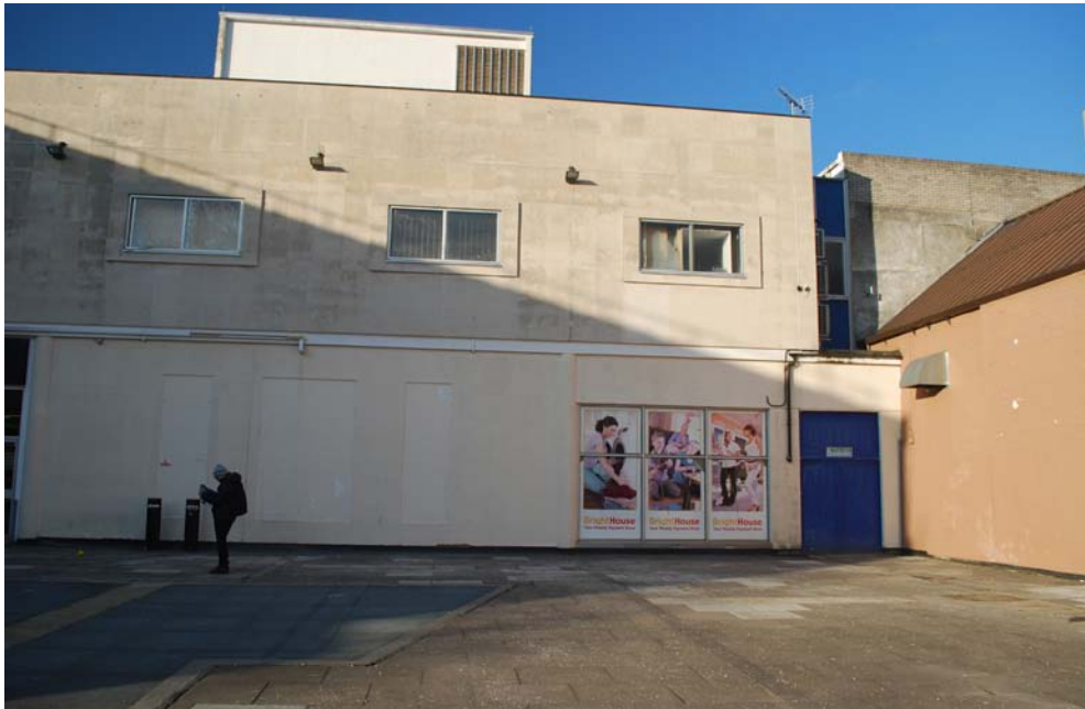
VIEW OF NORTH EAST CORNER OF SITE WITH FIRE EXIT
