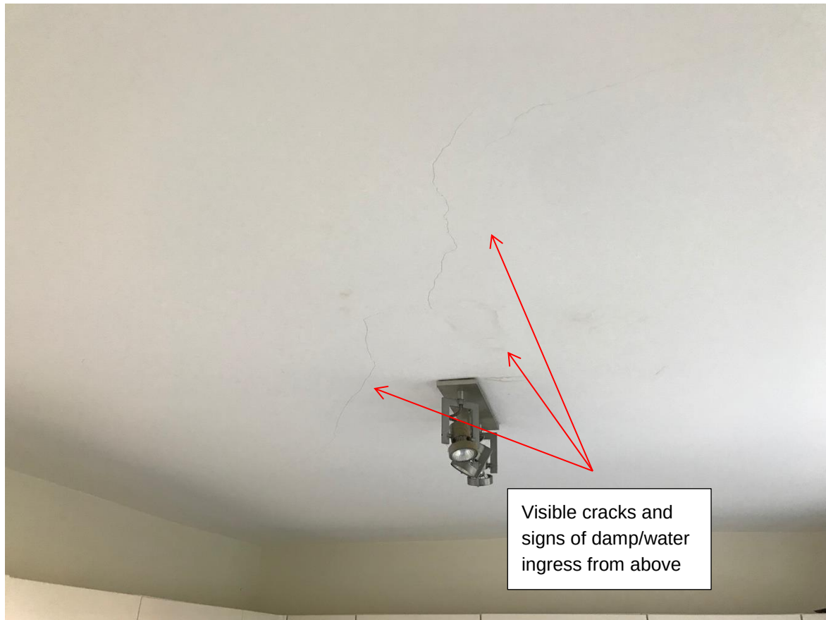
Figure 7: Kitchen/dining room existing ceiling
