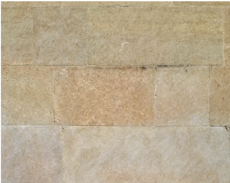
Ashlar Limestone external walls
