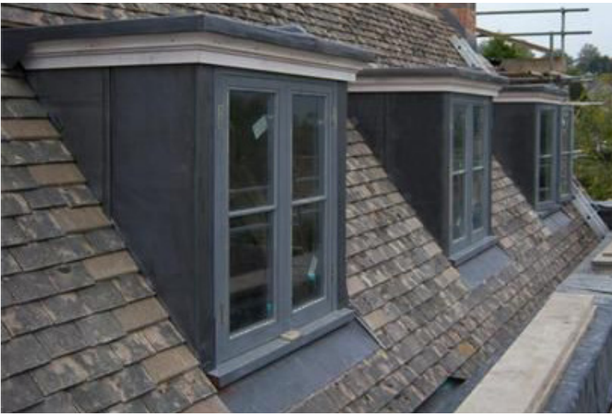
Lead dormer cladding
