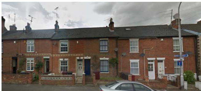
01 George Street - 2 storey with consistent fenestration
