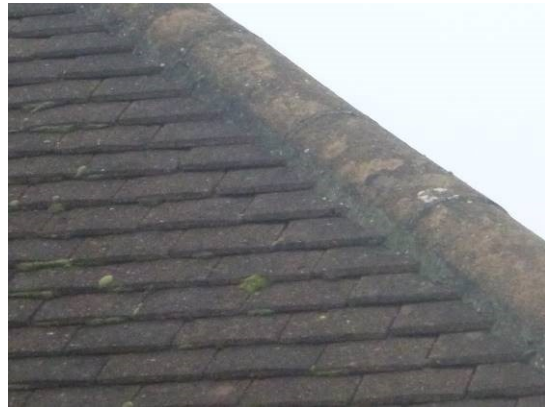
8. Hip tiles in place and fully mortared
