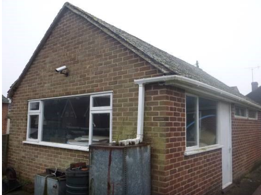
3. The pitched roof garage situated to the rear of the chalet bungalow
