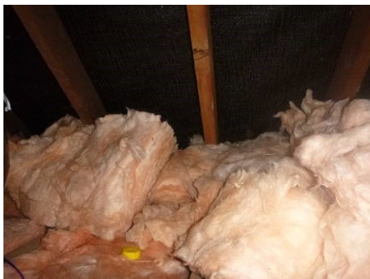
19. The roof space lined with bitumen felt.
