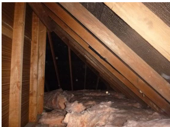
21. Internal view of the eaves space which was lined with bitumen felt.
