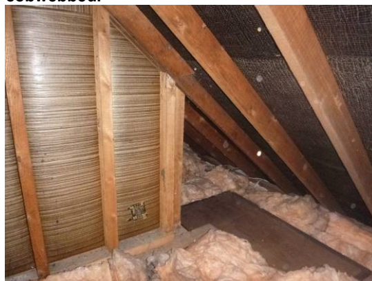
22. The internal walls of the eaves space insulated with fibreglass and paper.
