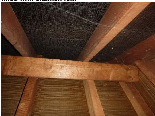
23. The cobwebbed rafters of the eaves space.
