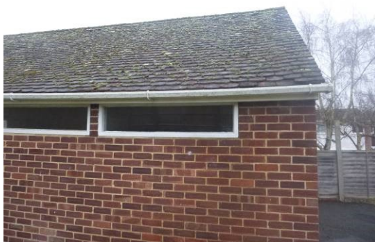
13. Roof tiles in place and tight on the garage
