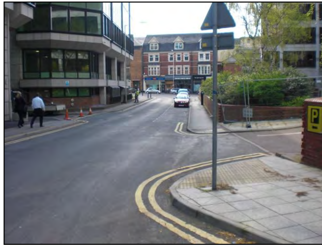
Figure 3 – Pedestrian crossing point at the car park access from Abbey Street
