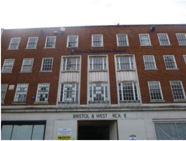
Plate 1. Exterior of 173-175 Friar Street - 'Bristol and West Arcade'
