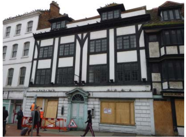
Plate 10. Exterior of 29-31 Market Place 'Coopers Arms'
