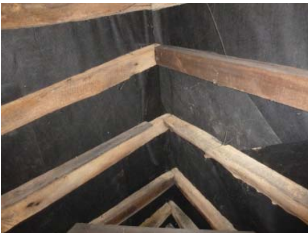
Plate 17. Bitumen lining of roof void of 29-31 Market Place 'Coopers Arms'
