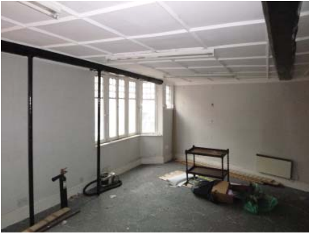
Plate 7. First floor of of 27-28 Market Place - 'Kik Sports'
