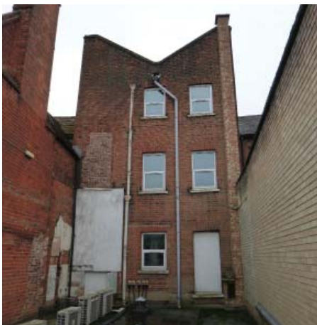
Plate 23. Rear exterior of 32 Market Place (interior of these levels not accessed during survey)
