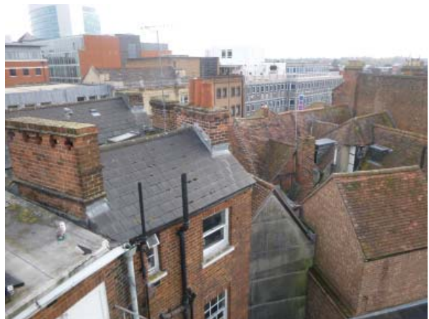
Plate 24. Roof structure of 27-32 Market Place
