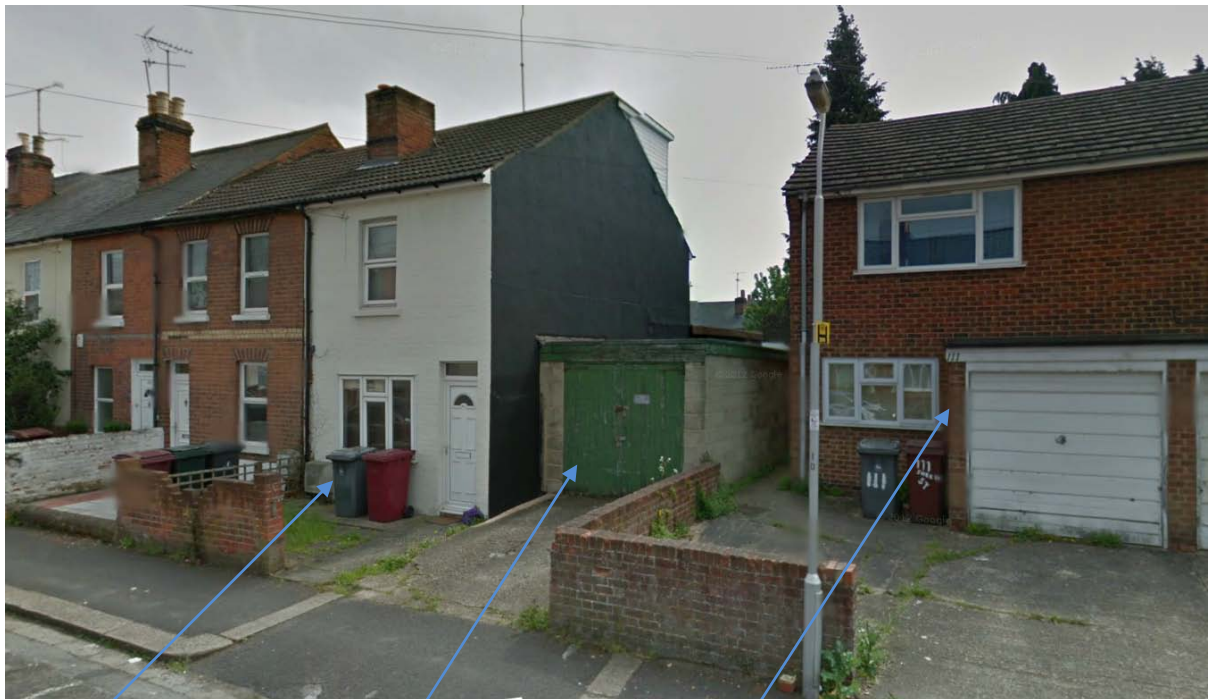
No 109 Garage plot No 111 Street view looking towards No 109 with the garage plot on the middle
