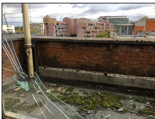
Figure 3: Parapet wall on eastern elevation of building on site
