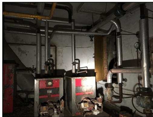
Figure 9: Interior of basement of the building on site
