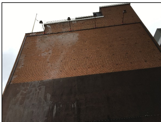
Figure 4: Northern elevation of building on site
