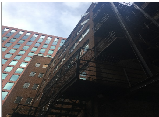
Figure 1: Western elevation of building on site
