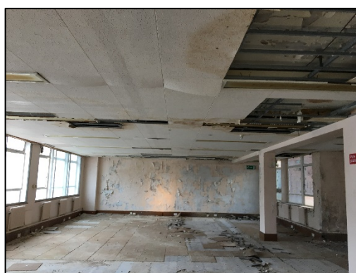
Figure 7: Interior of building
