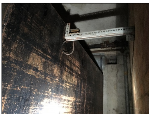
Figure 10: Inner room of the interior of the basement of the building on site
