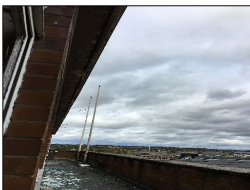
Figure 6: Lip of roof area with soffits
