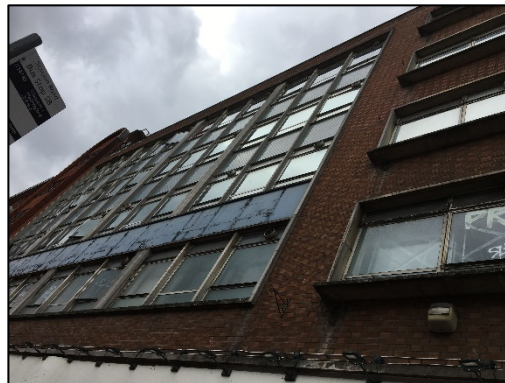
Figure 2: Eastern elevation of building on site
