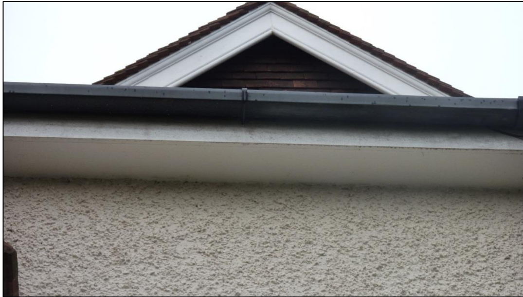
Photograph 5: Tightly fitted eaves
