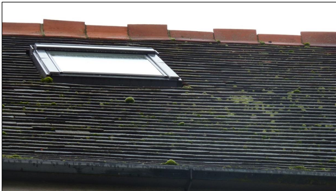
Photograph 4: Tightly fitted roof tiles
