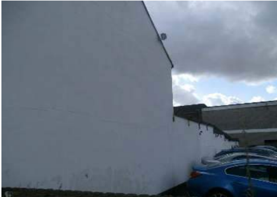
Looking at eastern boundary wall
