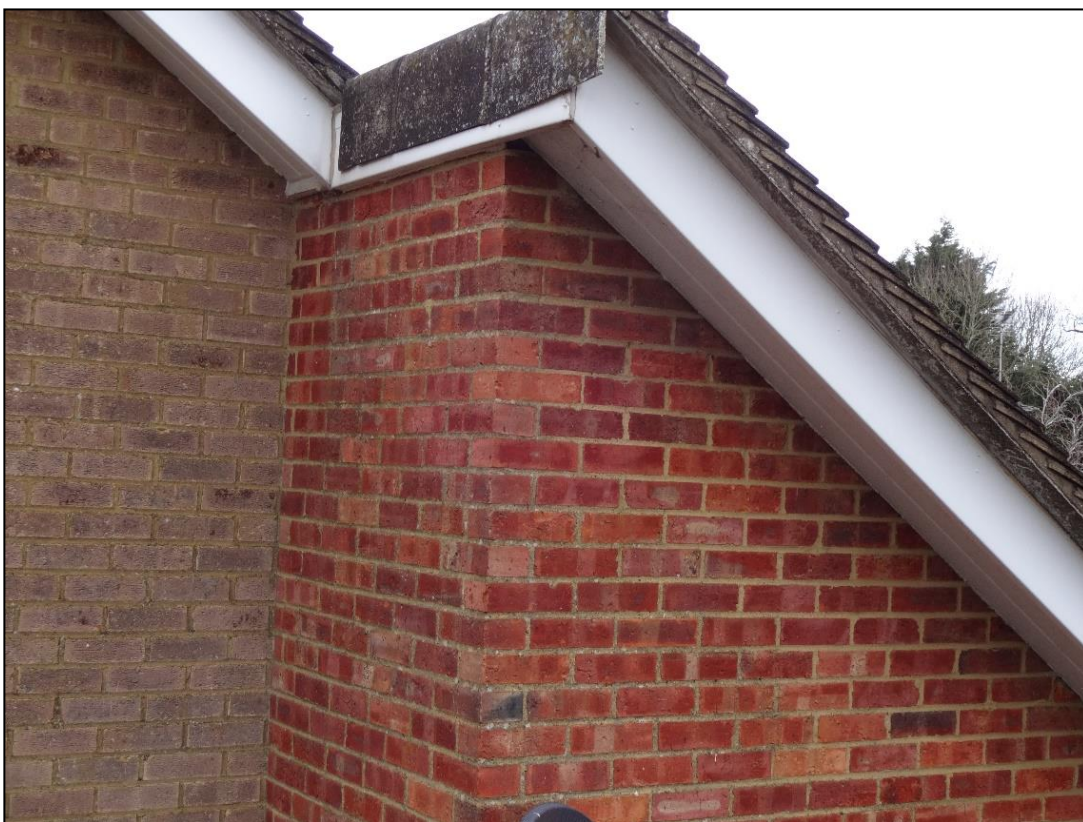
Figure 8. Close fitting uPVC fascias and soffits, 11 Yarnton Close, Emmer Green. 13.03.18
