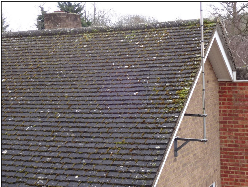
Figure 4. Close fitting roof and ridge tiles, 11 Yarnton Close, Emmer Green. 13.03.18
