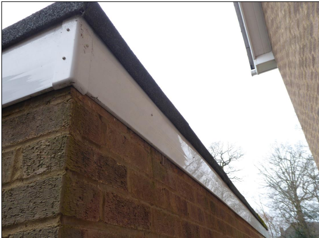
Figure 10. Close fitting bitumen and uPVC fascias on garage, 11 Yarnton Close, Emmer Green. 13.03.18
