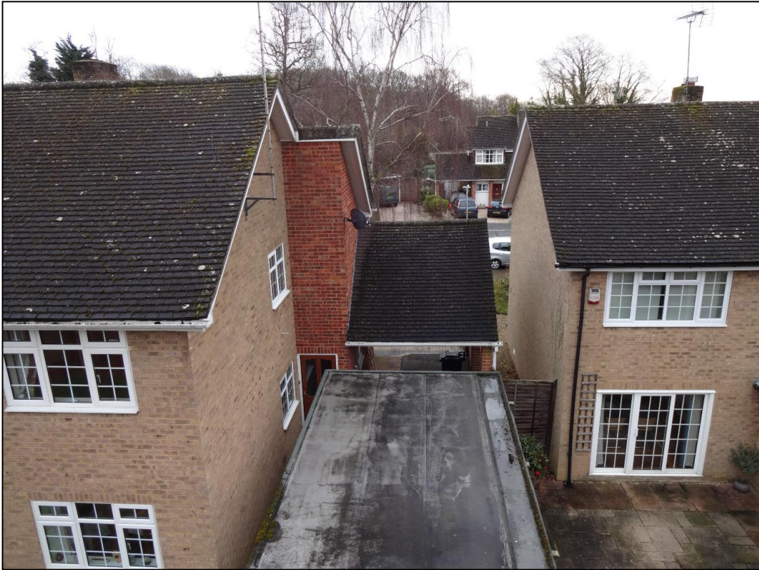
Figure 10. Close fitting bitumen and uPVC fascias on garage, 11 Yarnton Close, Emmer Green. 13.03.18
