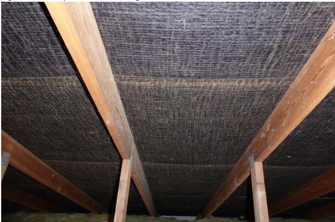
Figure 12. Example of bitumen lining. 11 Yarnton Close, Emmer Green. 13.03.18
