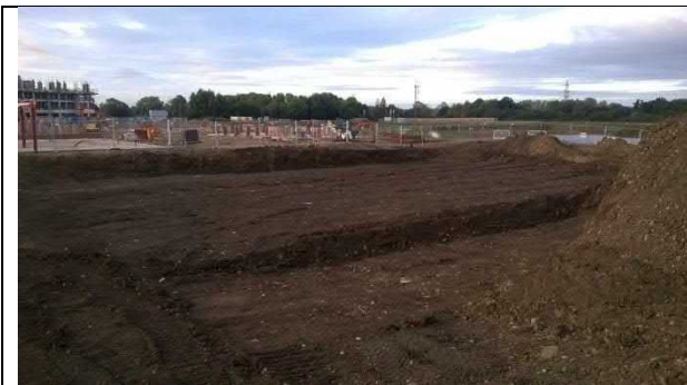
Plate 7 – Compaction of residual Made Ground
