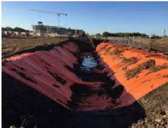
Plate 9 – Creation of clean service corridor
