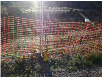
Background air monitoring during earthworks
