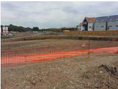
Example of air monitoring to west boundary of phase 5
