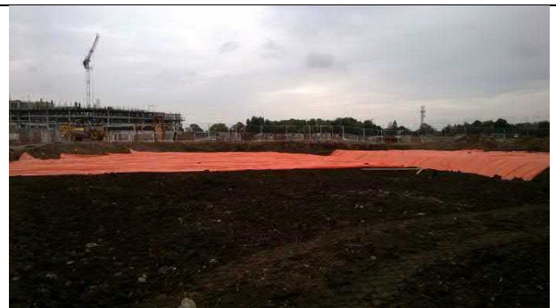
Plate 8 – Placement of orange marker layer
