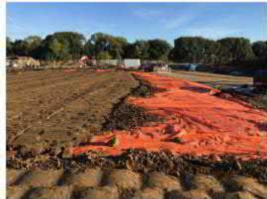
Plate 9 – Placement of orange marker layer
