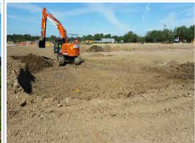
General works area photo
