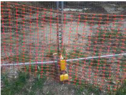
Background air monitoring during earthworks
