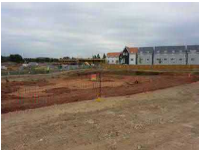
Additional example of air monitoring to boundary
