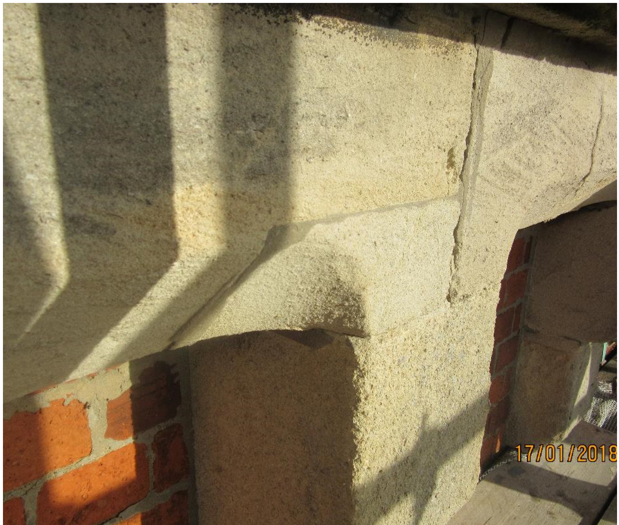
Photograph 8 - Repair to bathstone
