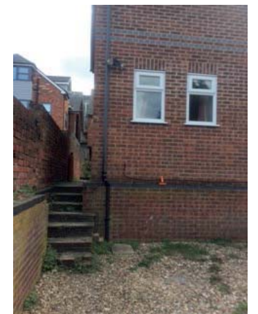
Building to the rear of 38-40 Crown Street - external steps up raised ground floor level
