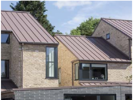
Pigmented metal standing seam roof on brick, Cambridge
