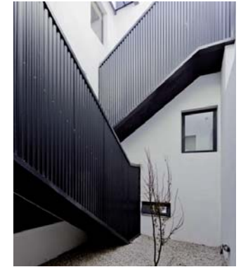
Staircase enclosed in grey corrugated metal, Hitzig Militello Arquitectos, Buenos Aires http://www.dezeen.com
