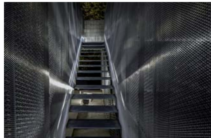
stair enclosed with metal mesh
