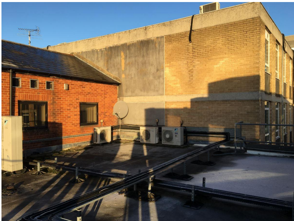
Roof level, looking towards the third storey of the building (left)
