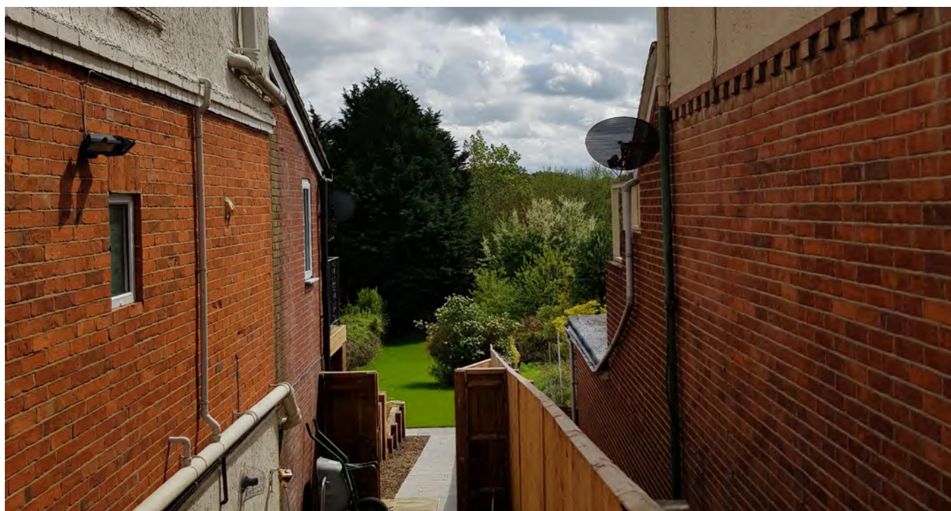
Photograph No. 16 - View of garden at the rear of B4 to which access was unavaivlable at the time of survey.
