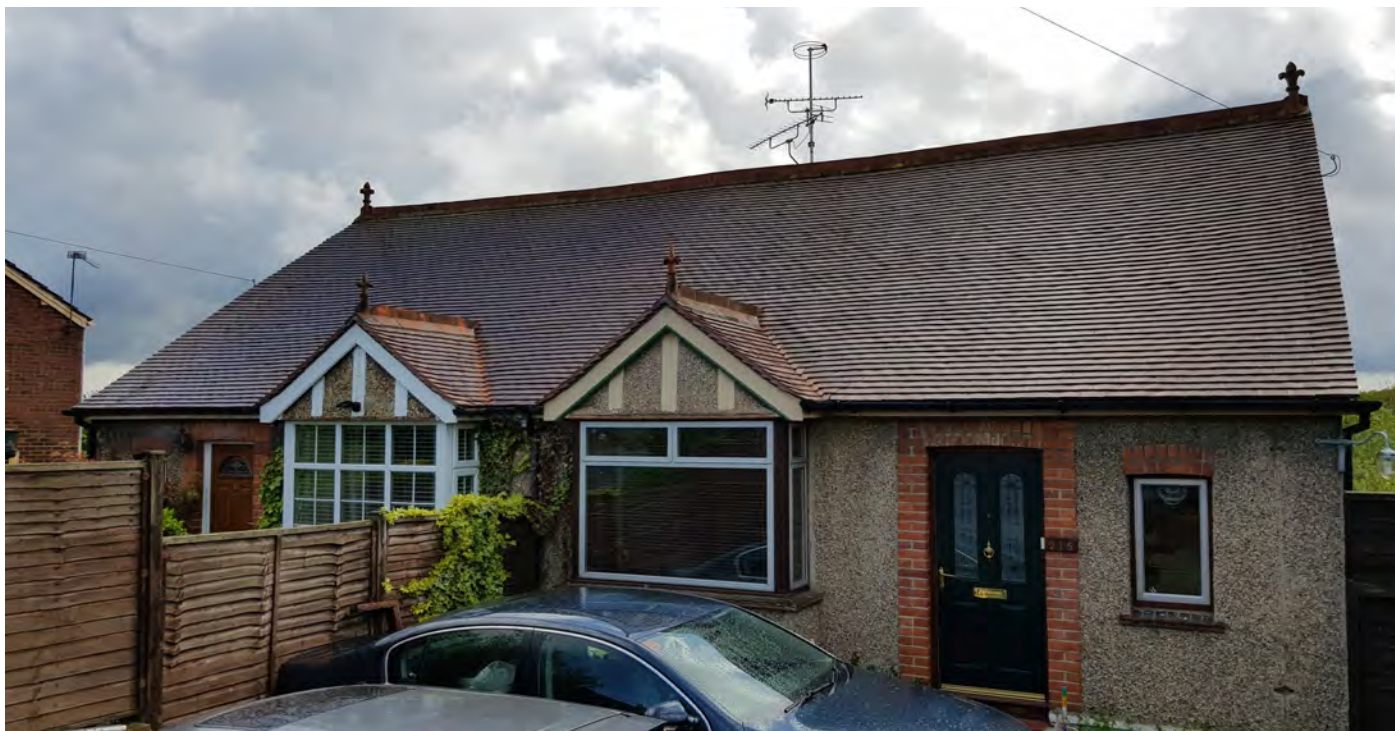
Photograph No. 5 - External View of building B2
