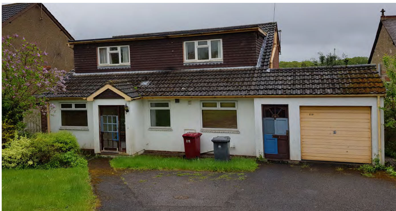
Photograph No. 2 - External view of Building B1.
