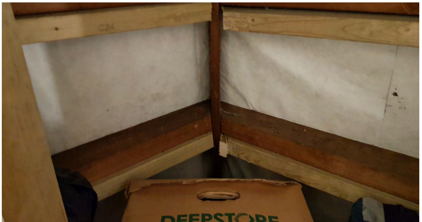
Photograph No. 10 - Internal view of Building B2.
