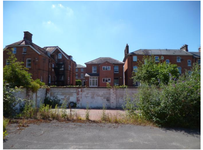
View of the rear of the Russell Street properties
