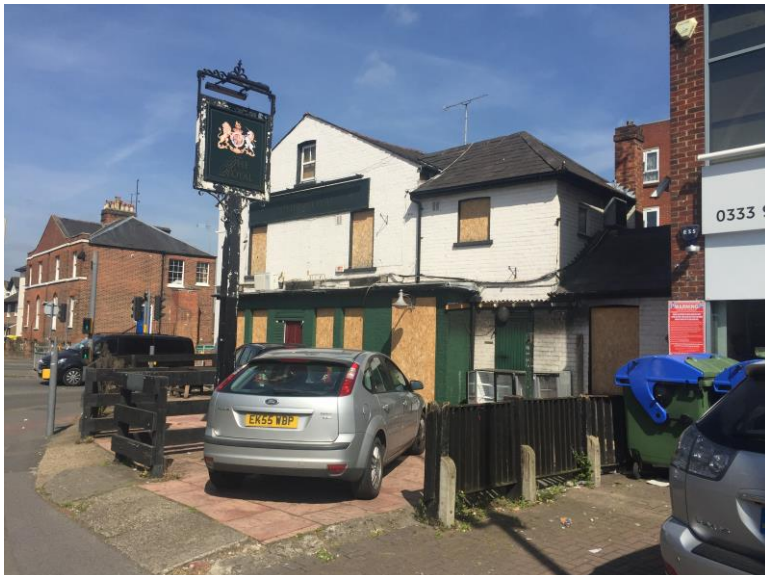
Figure 2 - Existing pub sign also showing individual external light Fittings fixed to the building
