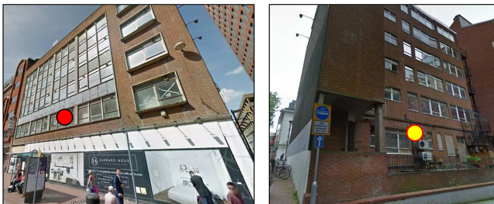
Figure 2.2. Noise survey location 1 at front façade (left picture) and location 2 to the rear façade (right picture) of the existing building on site.
