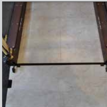
Special Floor Covering
