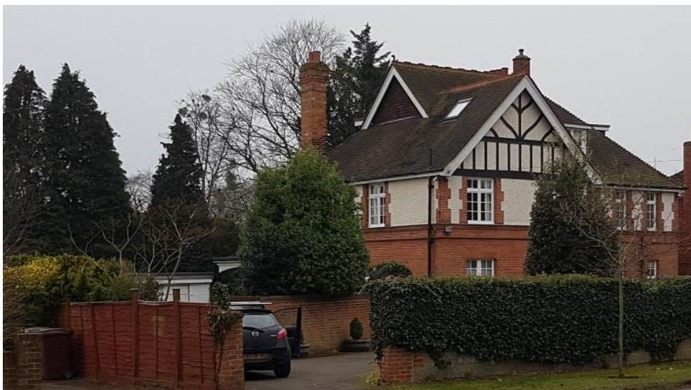
Figure 1: Existing house viewed from Grosvenor Road
