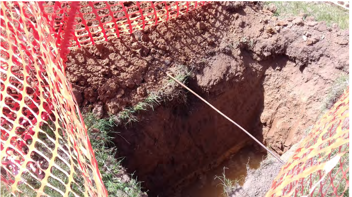
Above Trial Pit TP3
