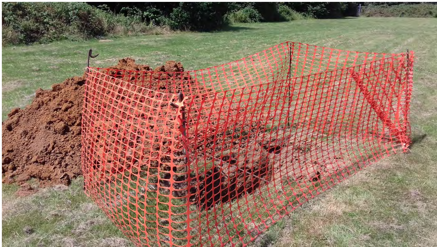
Above Trial Pit TP2
