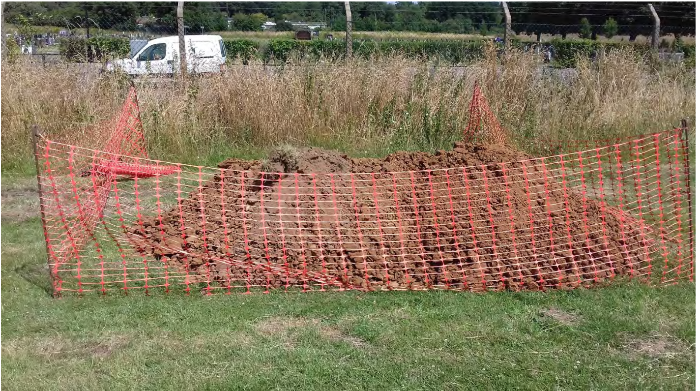
Above Trial Pit TP1
