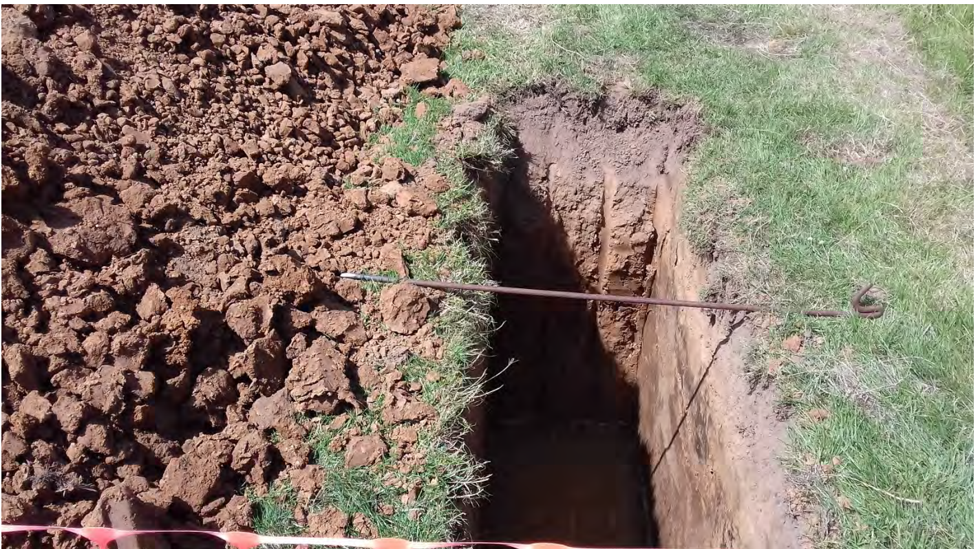
Above Trial Pit TP1
