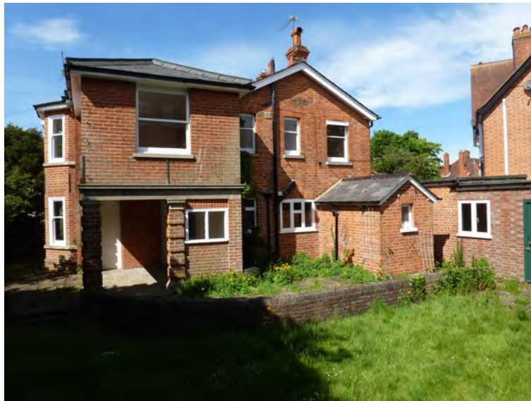
Fig. 2: Rear view of existing 25 Redlands Road
