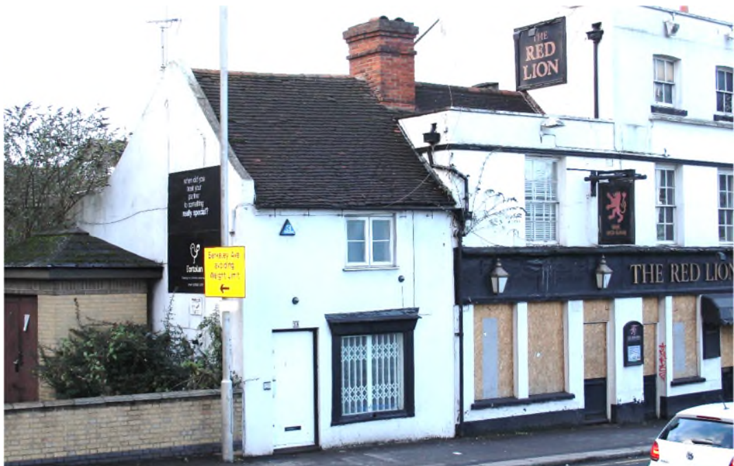
Figure 4 No. 38, front and south elevations.
