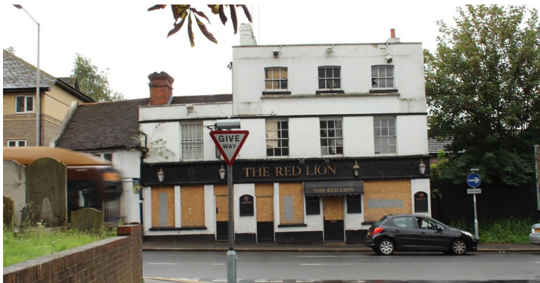
Figure 2 The former Red Lion, front elevation showing the two-storey element to the south of the principal block
