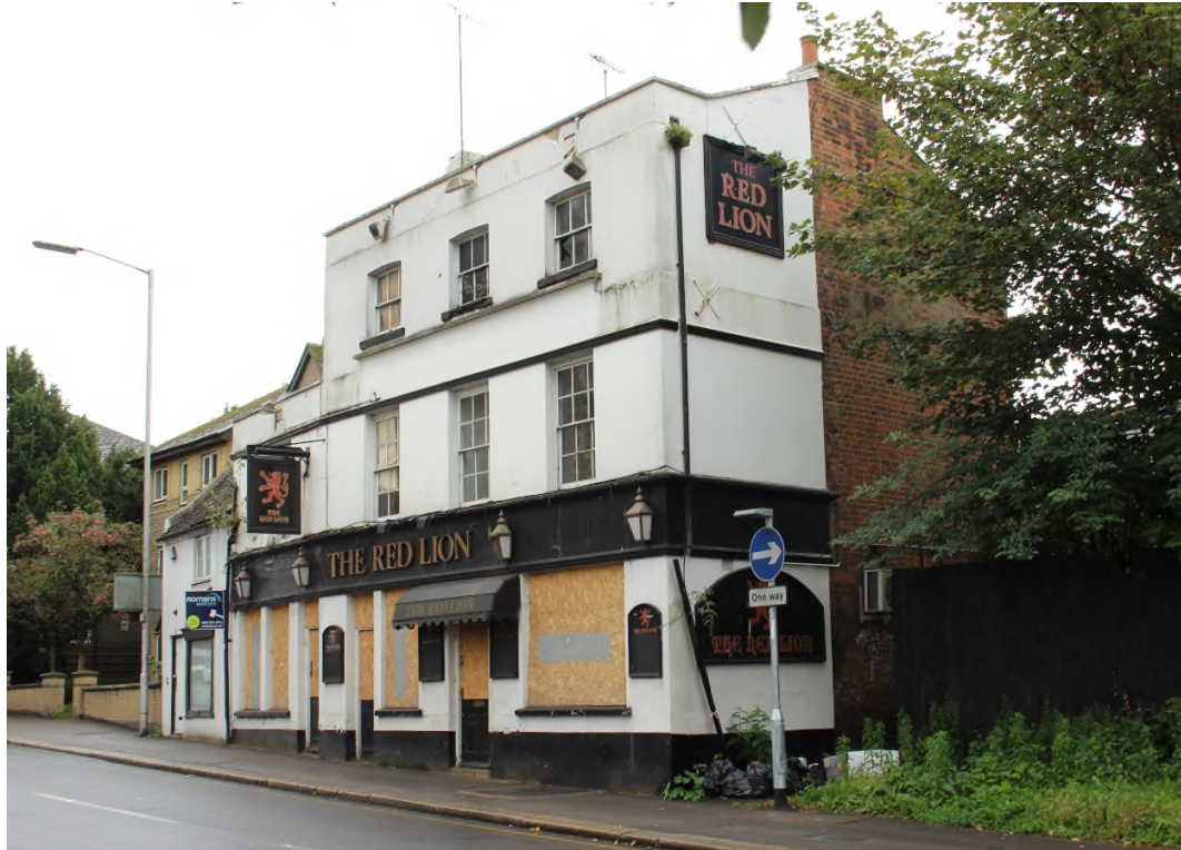
Figure 1 Front and north elevations
