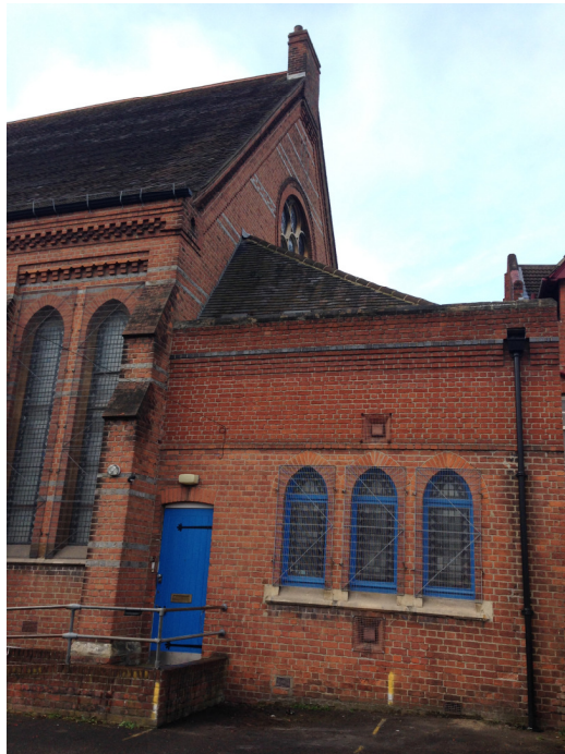
View from car park East side
