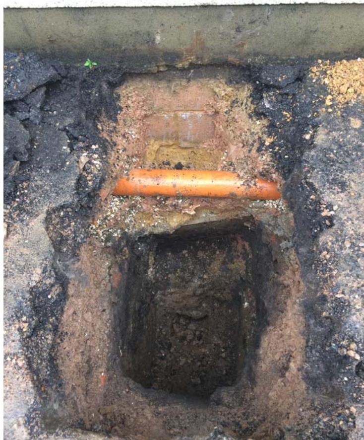
View of foundations and services encountered in Trial Pit No 1
