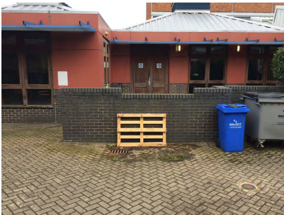
Photo 8 – Site of BH04, at right, to the west of the single storey element of the Engineering building.
