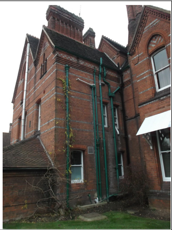
14) East Wing, Rear Elevation Two-Storey Projection.
