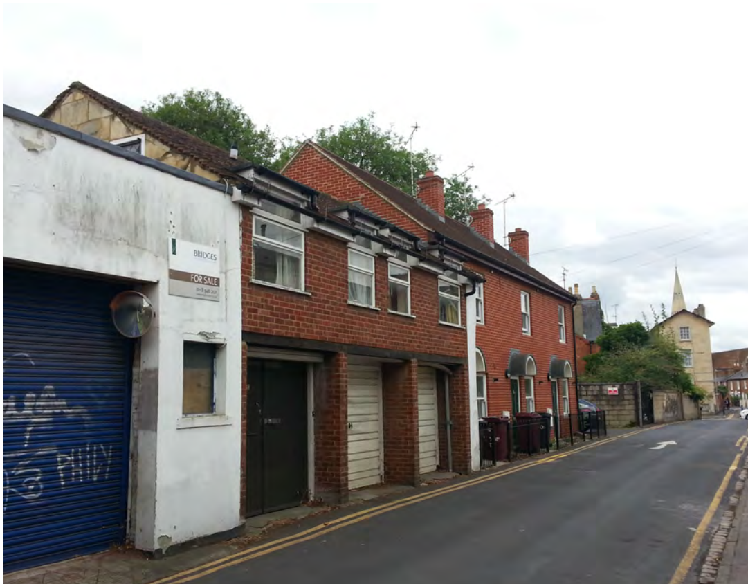
Fig.1: View of 12 Eldon Terrace from the street looking west
