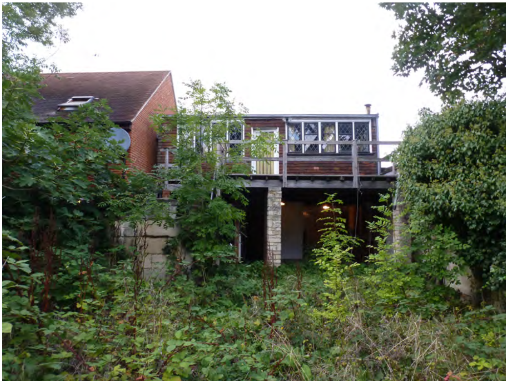
Fig.4: Rear view of 12 Eldon Terrace
