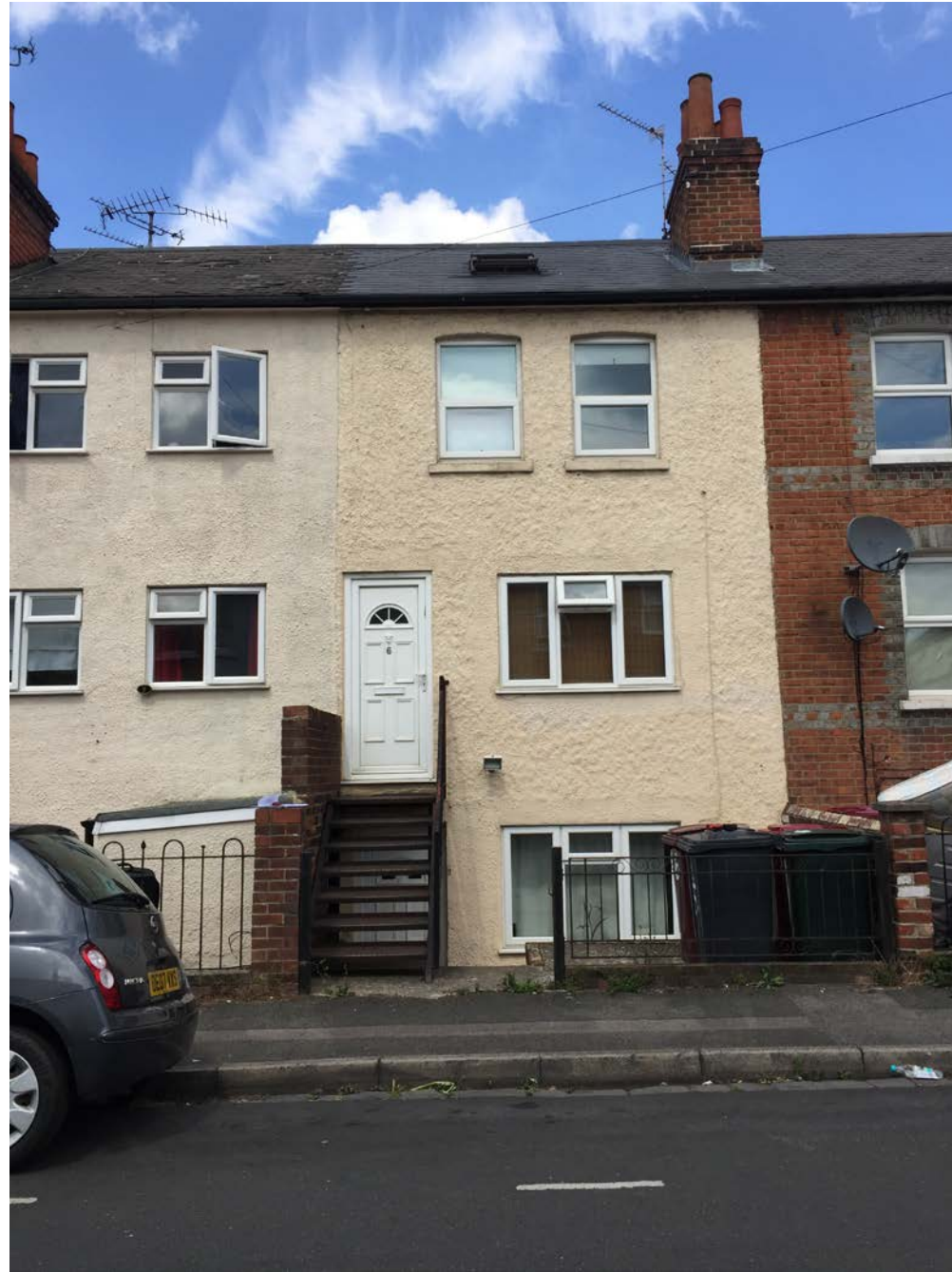
View from mason Street showing access and existing loft conversion
