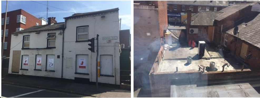
Figure 4 – The poor amenity for Number 10 Trinity Place. Left – The redundant public house is hoarded up. Right – The roofscape of the redundant public house.
