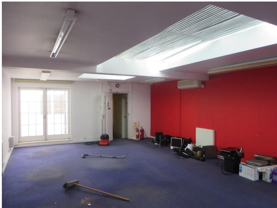
Rear extension -view toward lightwell and link to main building
