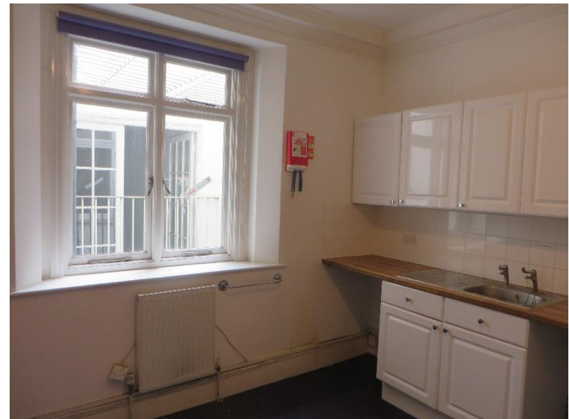
Ground floor rear of old building-modern window and typical skirting/ cornice details
