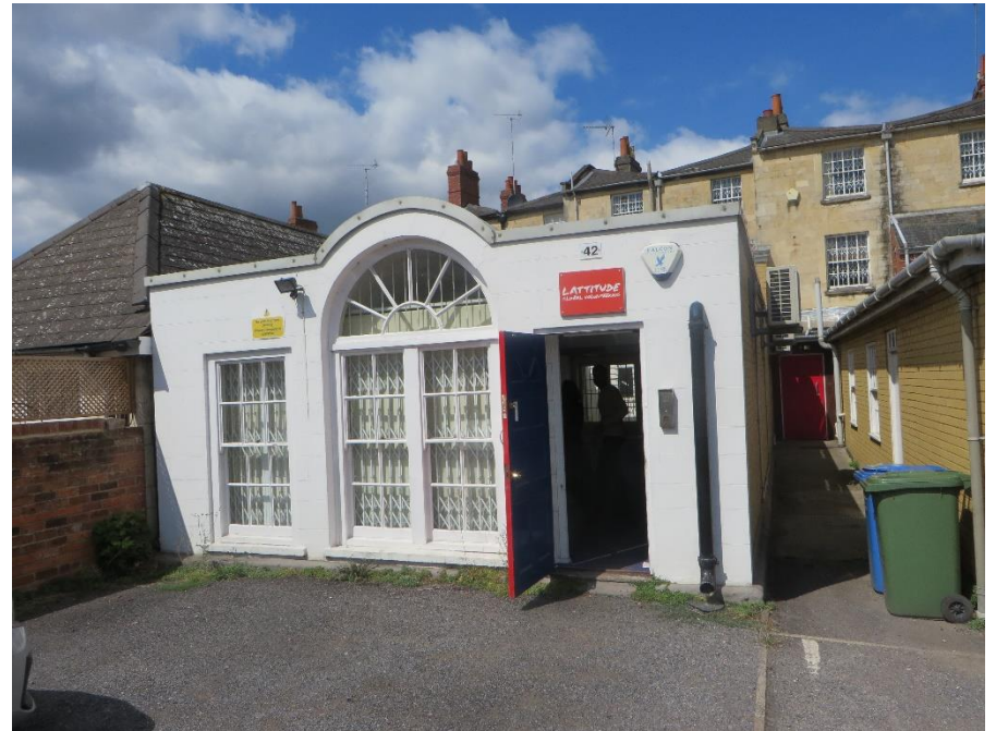
Rear extension seen from parking area
