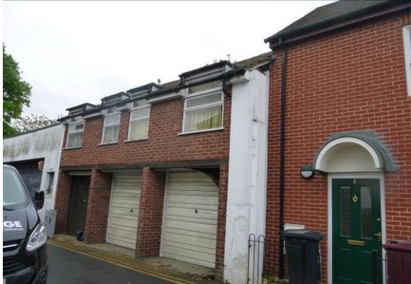
1. The front of the building viewed from the north west
