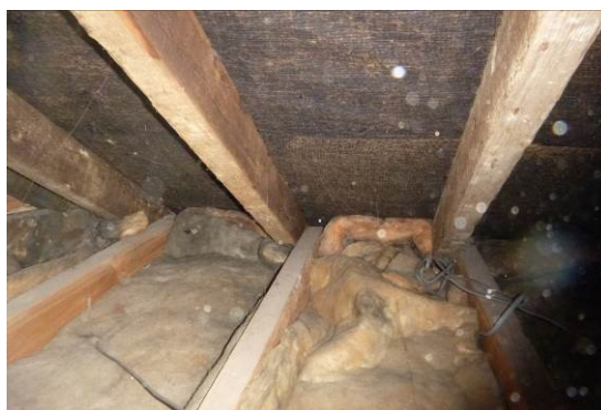
12. The fibreglass insulation tight to the eaves.
