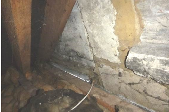
15. The eastern gable end and daylight in the corner into the room below.
