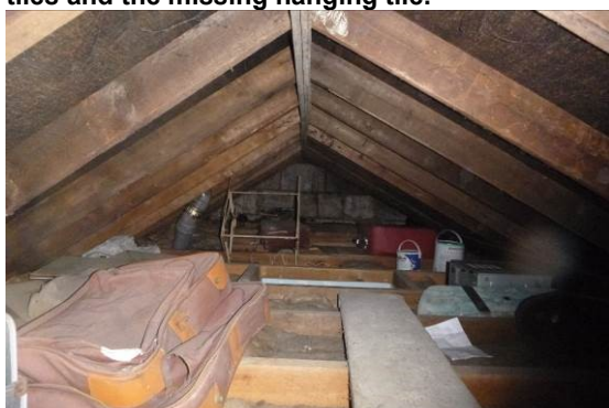
11. The roof space.
