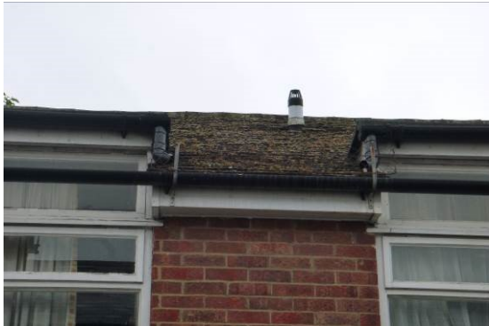
3. The tight flat roof tiles on the front elevation
