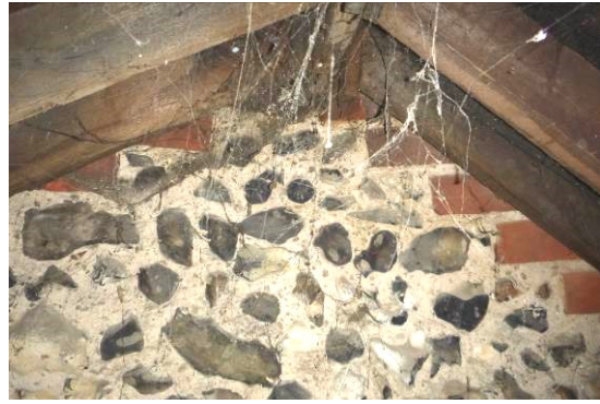
14. The western gable end.
