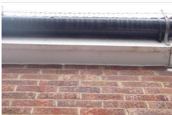
7. The tightly sealed soffit box on the front elevation.
