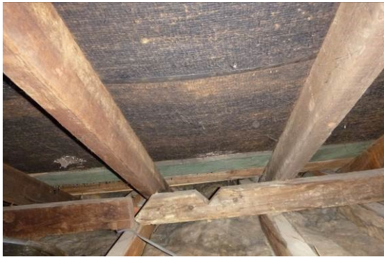
13. The eaves opening into the space in the flat roof.
