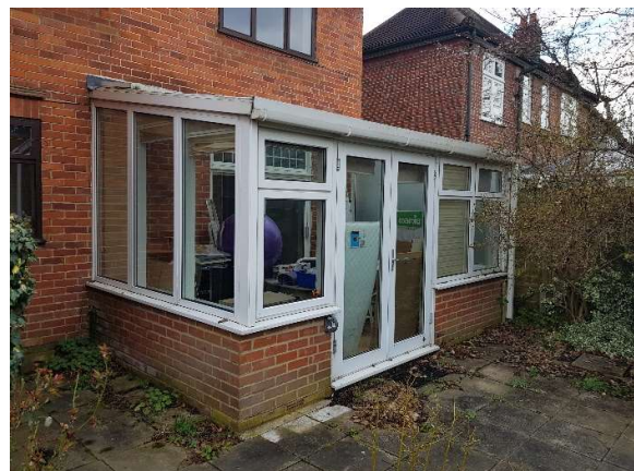
Figure 6: Existing Rear UPVC Conservatory
