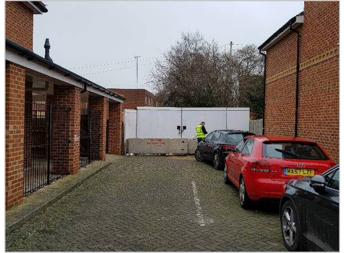
VIEW OF AREA 3 SITE ENTRANCE OFF VALENTIA ROAD
