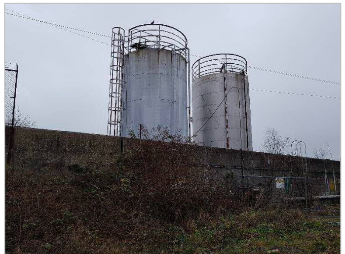
SILOS (NOTE: ONE CONTAINS CRUDE OIL, THE OTHER CONTAINED DIESEL BUT IS UNDERSTOOD TO NOW BE EMPTY)
