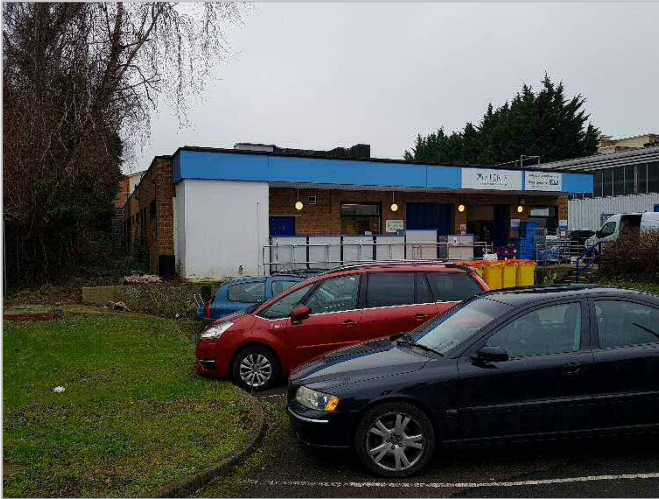
SYNERGY HEALTH BUILDING (NOTE: TO REMAIN OPERATIONAL THROUGHOUT CONSTRUCTION)
