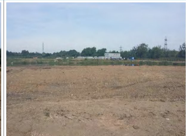
general works area photo
